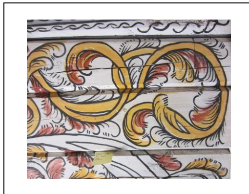
Figure 5. Old Stordal church, Norway. Detail from the south wall in the chancel. The yellow post-it note shows where the blue colour was observed and where the sample was taken. Photo: Tone Olstad©.
